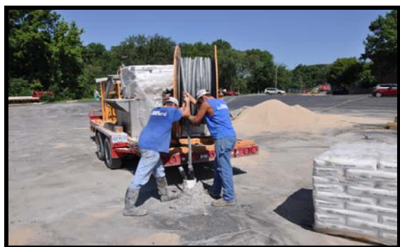
Crews pumping thermal grout into the wells.
