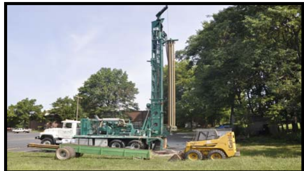
The drilling has started!
